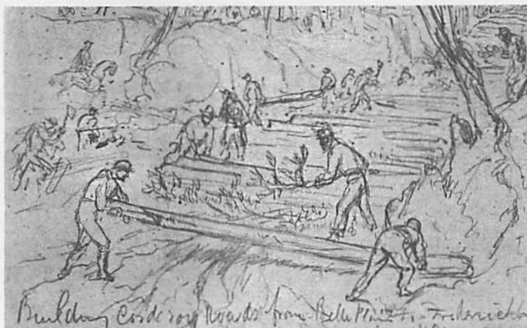
To make boggy roads passable for guns and wagons, men felled trees and laid the logs side by side across them to create a corduroy surface.
