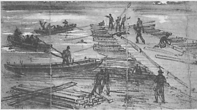
Union engineers, here building a pontoon bridge at Fredericksburg, were targets for sharpshooters, whom Longstreet called Confederate hornets.
